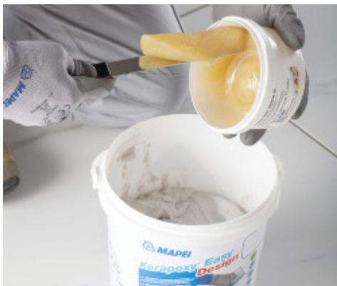
Pour the hardener (component B) in the container of component A
